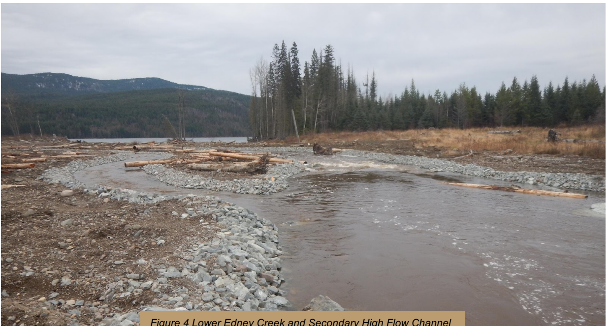
Figure 4 Lower Edney Creek and Secondary High Flow Channel
