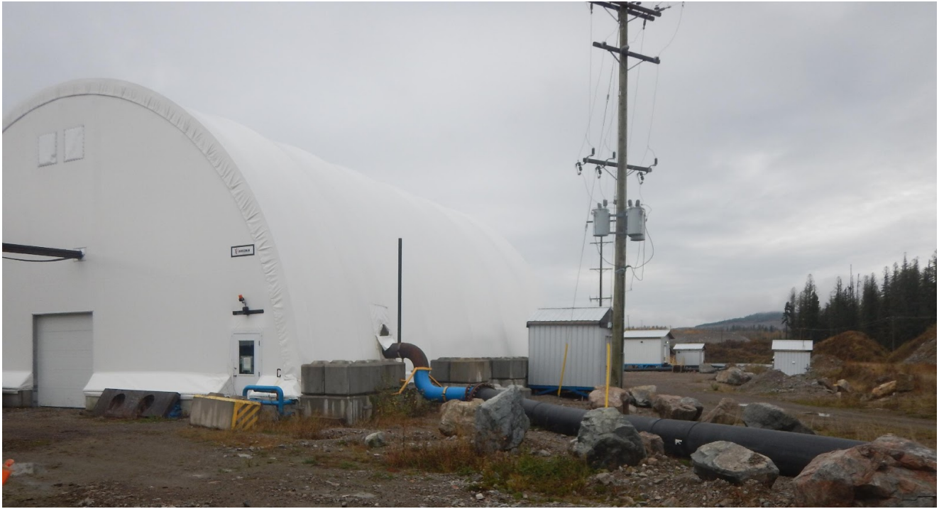
Figure 3 Water Treatment Plant and Discharge Pipeline to Quesnel Lake
